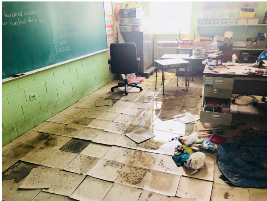
*THIS CLASSROOM SUSTAINED WATER DAMAGE FROM HURRICANES IRMA AND MARIA, CAUSING MOLD AND MILDEW IN ITS FLOORS AND WALLS.*
