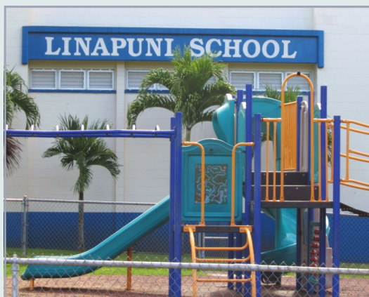
Source: OIG photo
